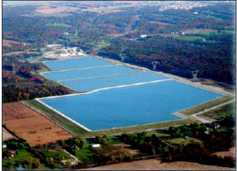
Del-Co Water Headquarters and Up-Ground Reservoirs on State Route 315, Liberty Township. The newest addition is the 1-billion-gallon reservoir at the bottom of the photo. Source: BBC&ME Engineering
